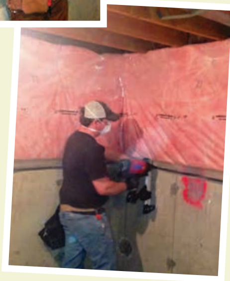
EnviroCentre staff insulating basement wall and header.
